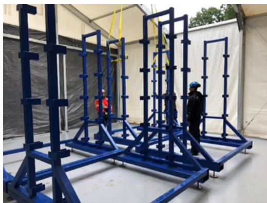
The site at Dansk Salt in an early phase of the commissioning
